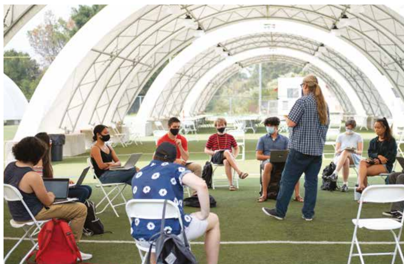
Saint Mary’s College of California constructed 12 pavilions to move in-person classes outdoors during the pandemic.
